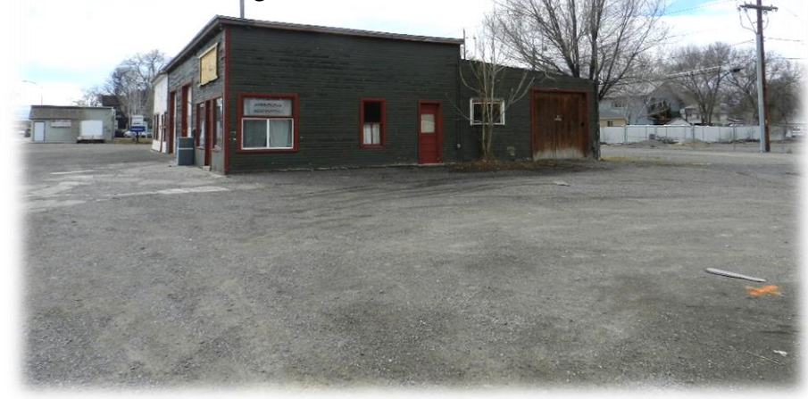
East side of building
