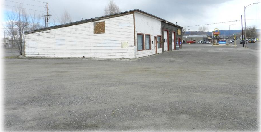
West side of building
