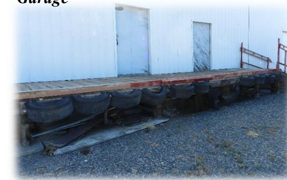
3' high loading dock with ramp
