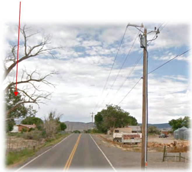
3-phase power line
