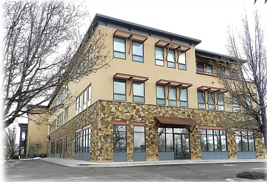
West Side of Building
