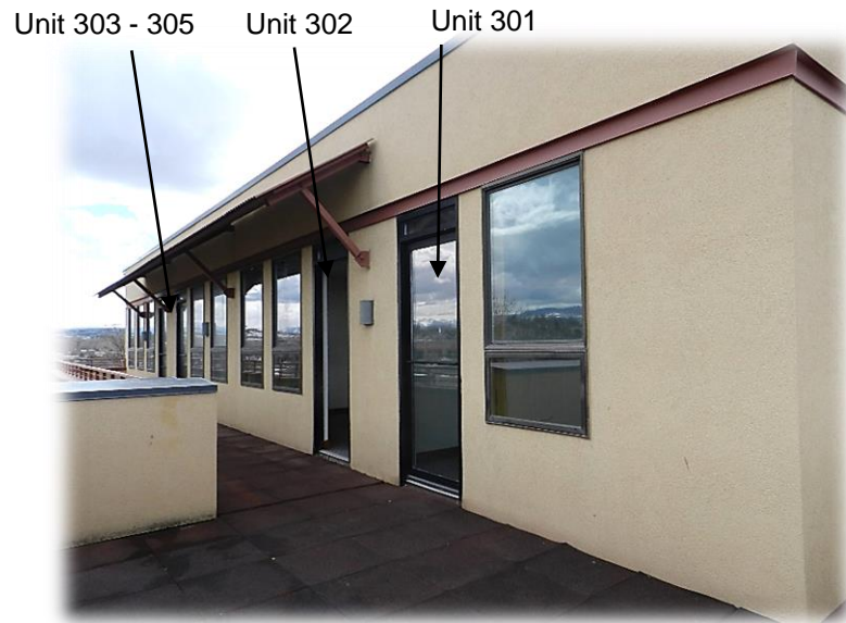
Balcony From Units 301, 302, & 303 - 305, Facing S Townsend Ave
