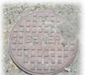
8" sewer main & tap installed. Sewer line inside the development is owned by the developer
