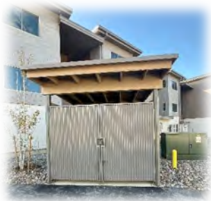
Enclosed shared trash dumpster
