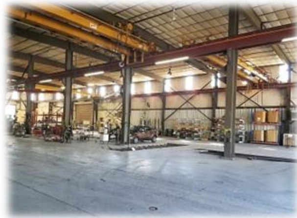
Main Fab Shop (Looking Southeast) North 5-Ton Overhead Crane
