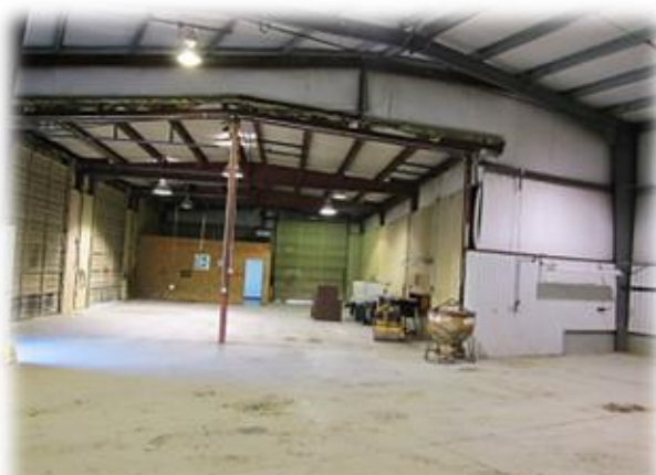
Maintenance Shop (Looking South)
