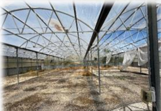
Partially finished Greenhouses
