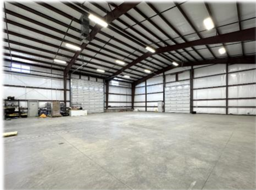
A-6 – South Side of Building A
