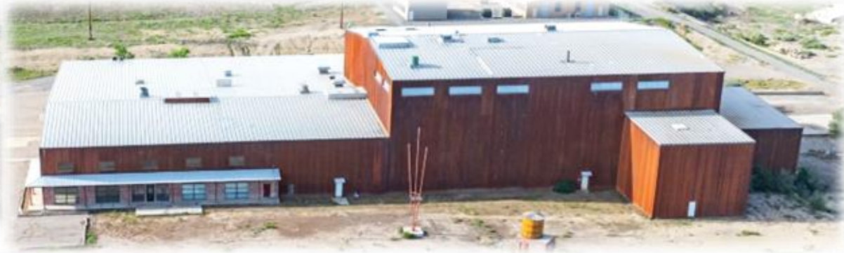
View of Facility facing North/Side Entrance
