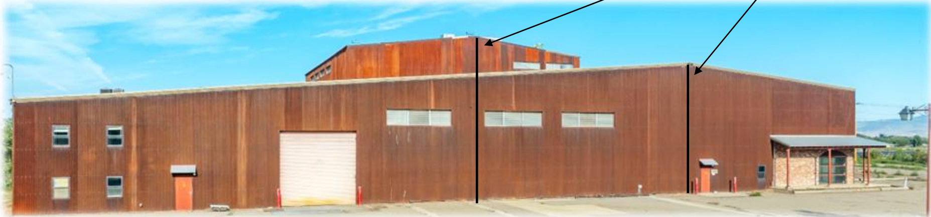
View of Facility facing West/Front Entrance
