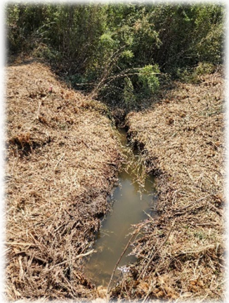
Ditch entrance onto the property
