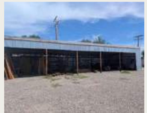
Covered storage at the rear
