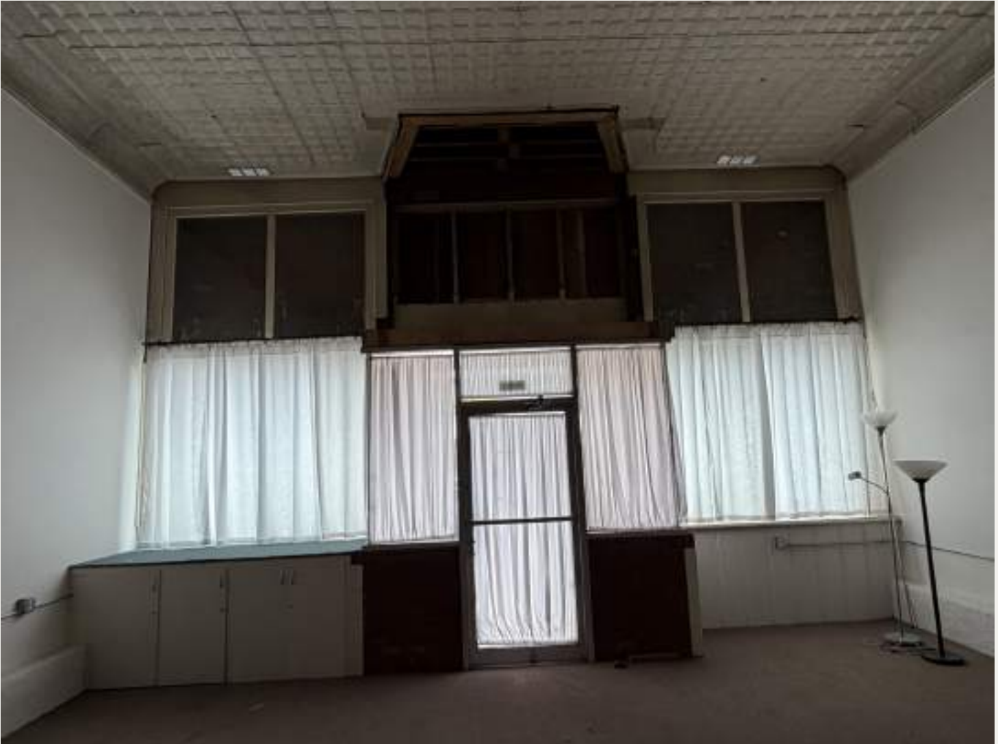
Retail storefront from inside: door and windows, ceiling to floor. 14± ft tin ceiling; remodeling has started and is to be completed.
